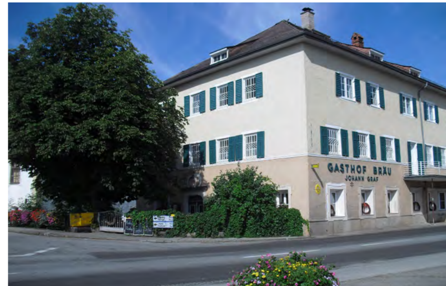
The Braeu, a formerly vacant inn that now houses a restaurant, co-working space and seminar house. ©Energie Munderfing
